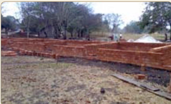
Building new dormitories, Inhaminga
